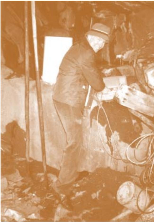
*Jason installing seismic station “#21” in Fagurholsymri, Iceland, July 2, 1996.*
